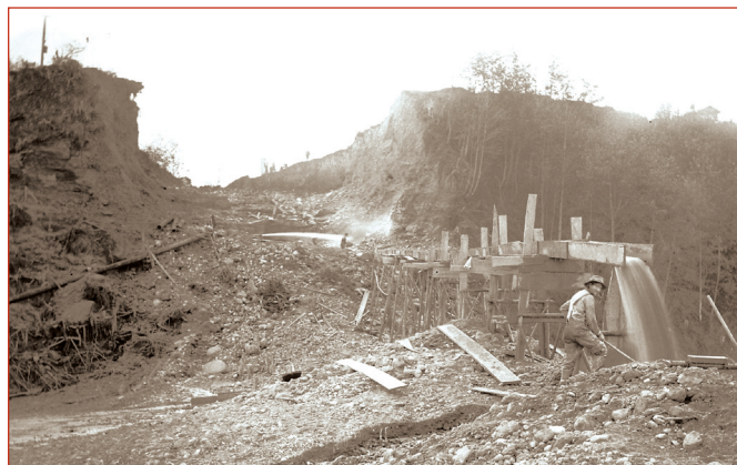
Sluicing the hill took a lot of hard work using a hand shovel. Photo ca. 1914.
