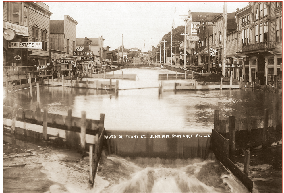
Water cascades over dams built to manage heavy mud flows during the sluicing project. (photo circa 1914)
