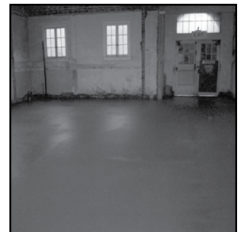
Gleaming new floors complete replacements.
