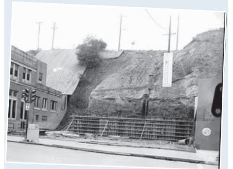
Creating the retaining wall and the fountain area. Stair will angle around behind the wall.
