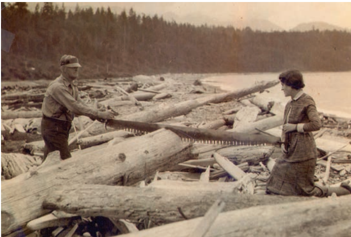
Adelbert Smith and daughter Opal cutting log ends to be used in the Lodge they were constructing for The Place Resort. Looking west near the mouth of the Elwha River, ca 1928.
